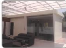
Green House Ventures, Pune
